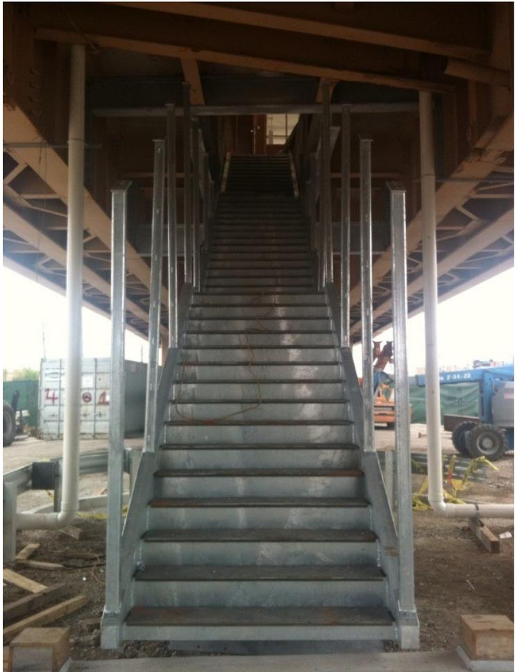
**Structural steel in place for new staircase to platform and walkway to stationhouse.**
